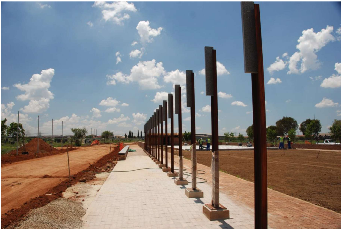
Construction of the Sharpeville Memorial – Photo credits (SACLAP ARCHIVES)
